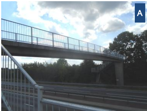
Bridge over A34
